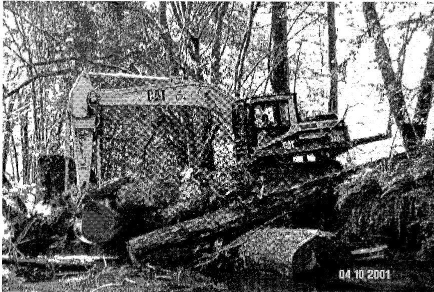
Figure 19. Placement of large wood in the Little North Fork of the Gualala River. Photo provided by Henry Alden, Gualala Redwoods, Inc.
